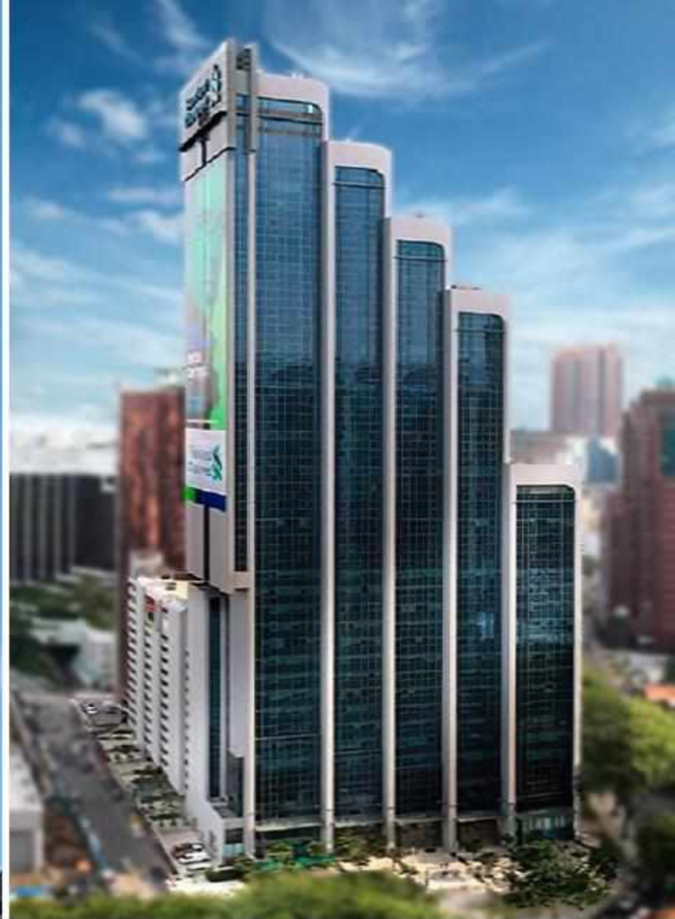
Menara AIA Sentral, Kuala Lumpur
