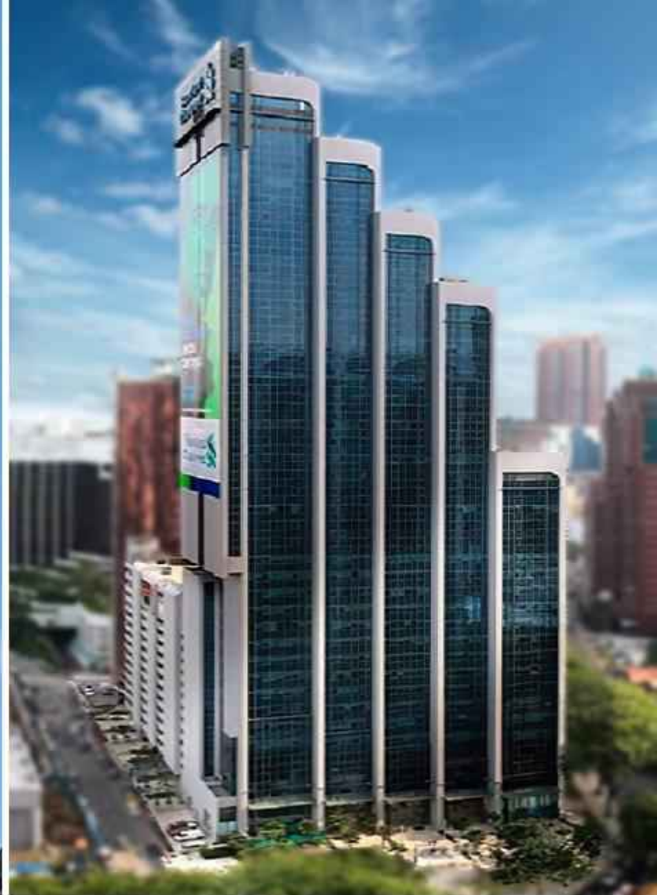
Menara AIA Sentral, Kuala Lumpur
