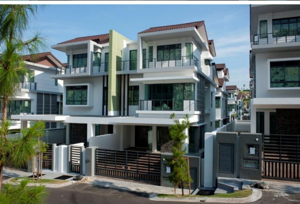
The Setia Pearl Island project is an environmentally sustainable Semi-detached housing project for SP Setia Berhad located in the highlands of Penang.
