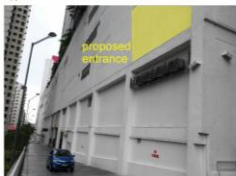
Proposed entrance into Glo mall. The pedestrian bridge shall be built between the building and boundary wall next lot which has a gap of approx. 8 feet. The entrance shall discharge directly to the first floor of the mall.
