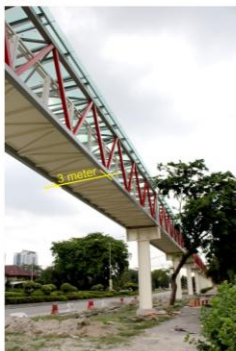
Pedestrian bridge built by Sunway linking the major buildings around the area. The bridge is a light weight steel truss system, supported by single steel columns in tight spaces. Pedestrian walkway is 3 meter, hand-rail to hand-rail.
