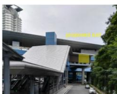
Proposed direct exit from station after checking out without changing in levels. The proposed exit is approx. 10 meter above road level.
